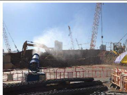
Regularly water spraying at the stockpile and keep the pathway of transferring stockpile moist
